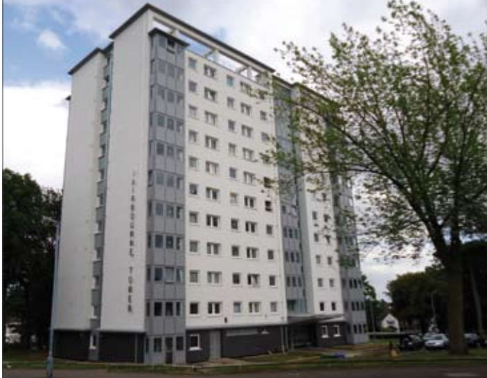
Fairbourne Tower After Refurbishment
