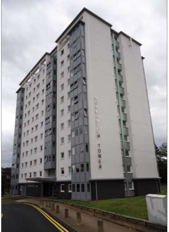
Normanton Tower After Refurbishment
